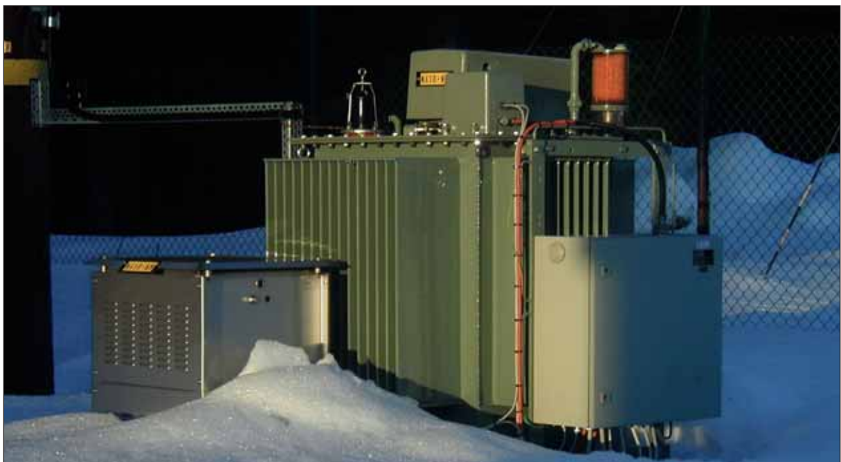
Fig. 3 10 kV Arc suppression coil
