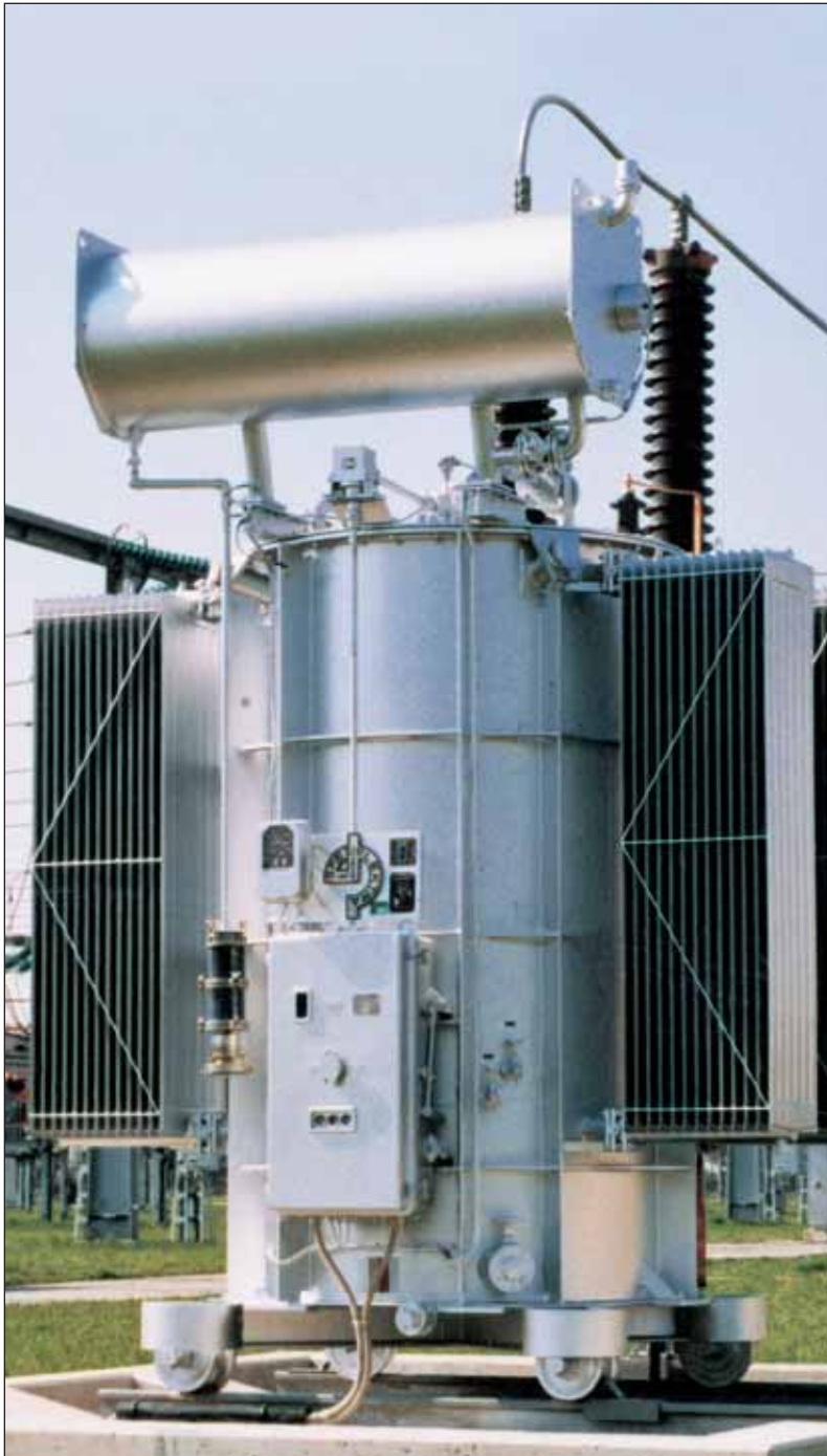
Fig. 4 110\sqrt{3} kV, 8000 kVar, continuous duty
